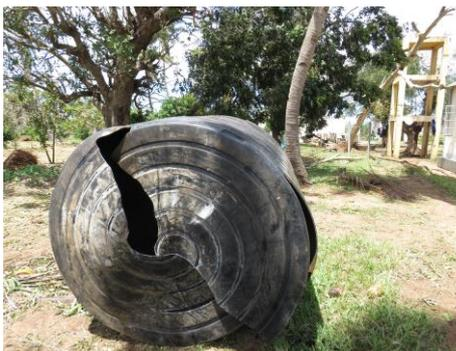
*The fall of a tree (top right) has damaged the elevated tank (Maxixe primary school)*
