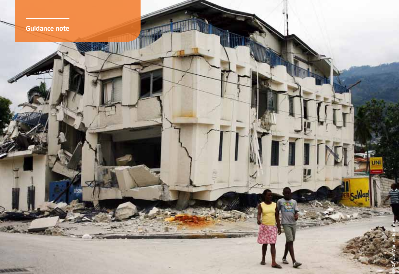
People walk by damaged buildings in Port-au-Prince, Haiti after the devastating 2010 earthquake.
