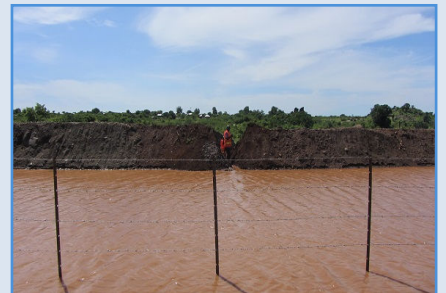
Flooded sections of the internal and external road after the rain on 21 May—PoC3, Juba
