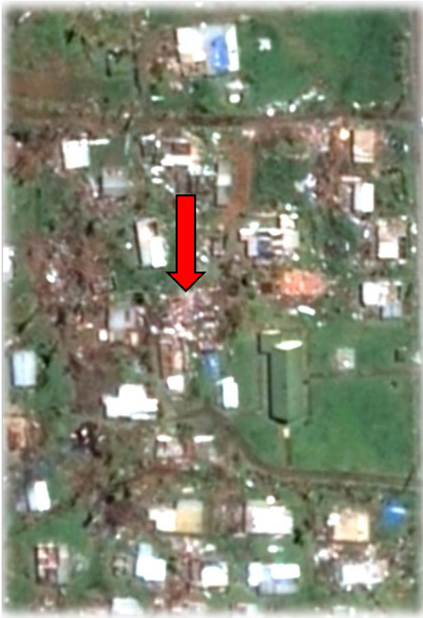
Post-Event-Image – Damaged Houses
