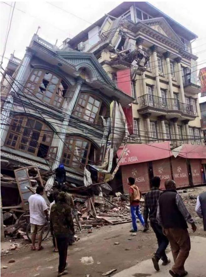
Photo 1: Building tilted due to earthquake in Nepal
