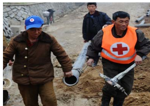
Construction of water supply system in target community. Photo: IFRC
