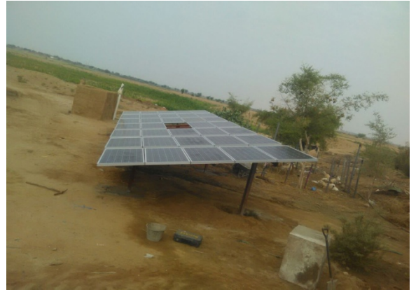
3 - Solar Water Pump Installed .
