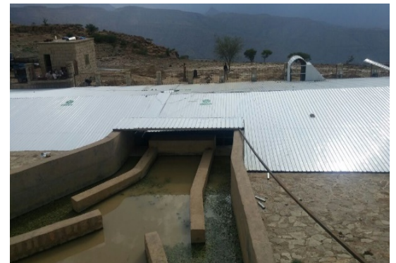
Figure 2 Rain Water harvesting roof - Khamir
