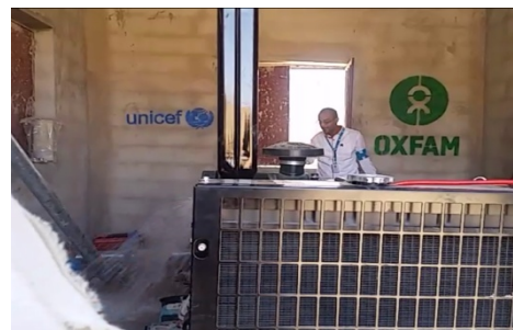
Figure 3 - Water pump installation - Amran
