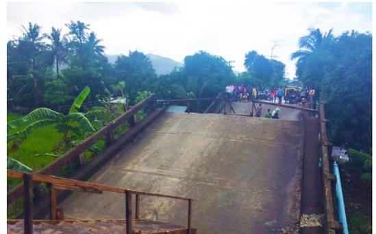
Credit: OCHA/M. Malang San Francisco, Surigao del Norte (14 February 2017) - The Anaon Bridge split into three places during the earthquake, cutting off access to Surigao City. Vehicles are crossing a river as a detour, which may be impassable during heavy rains.
