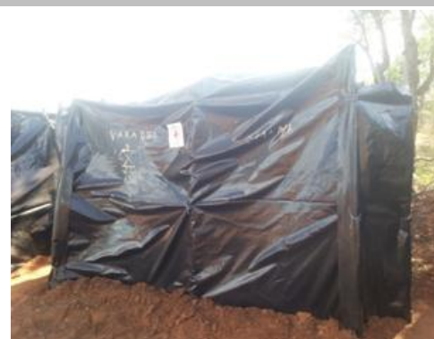
The temporary latrines established by ZRCS. Photo: ZRCS
