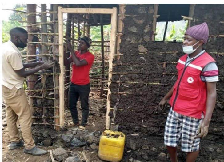
Building emergency shelters using mud and sticks ©RRCS
