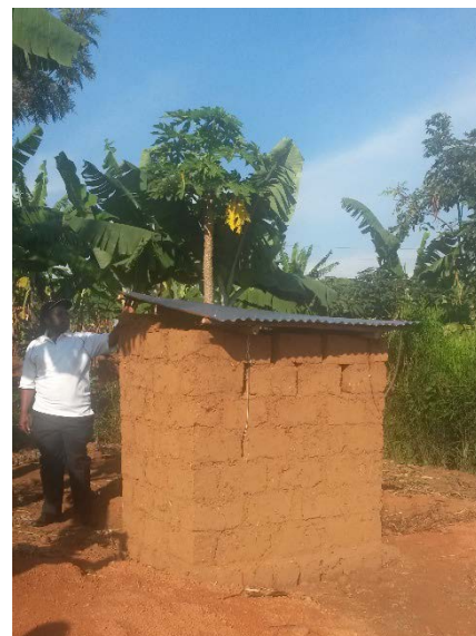
Community leader inspects one of the roofed latrines ©IFRC
