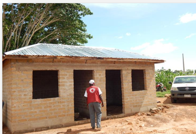
Shelter construction in Adamawa, in Hong Community. Photo NRC
