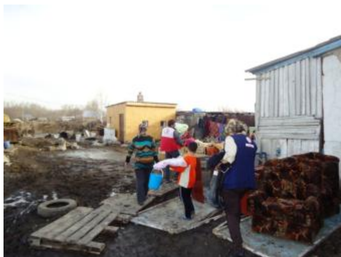
Cleaning operation after the flash flood. Photo: Kazakh RC
