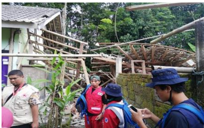
PMI volunteers are assessing damage in East Lombok. (Photo: PMI)
