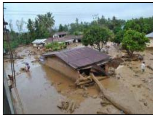
Caption: A house was damaged by the logs brought by the flash flood in Aceh Tenggara. Courtesy: http://www.tribunnews.com/2012/04/15/5-warga-lukaringan-akibat-banjir-bandang-aceh-tenggara
