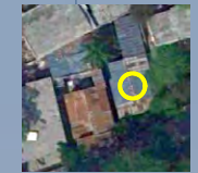
GRADE 1: NO VISIBLE DAMAGE ; Assessed building does not appear to be damaged
