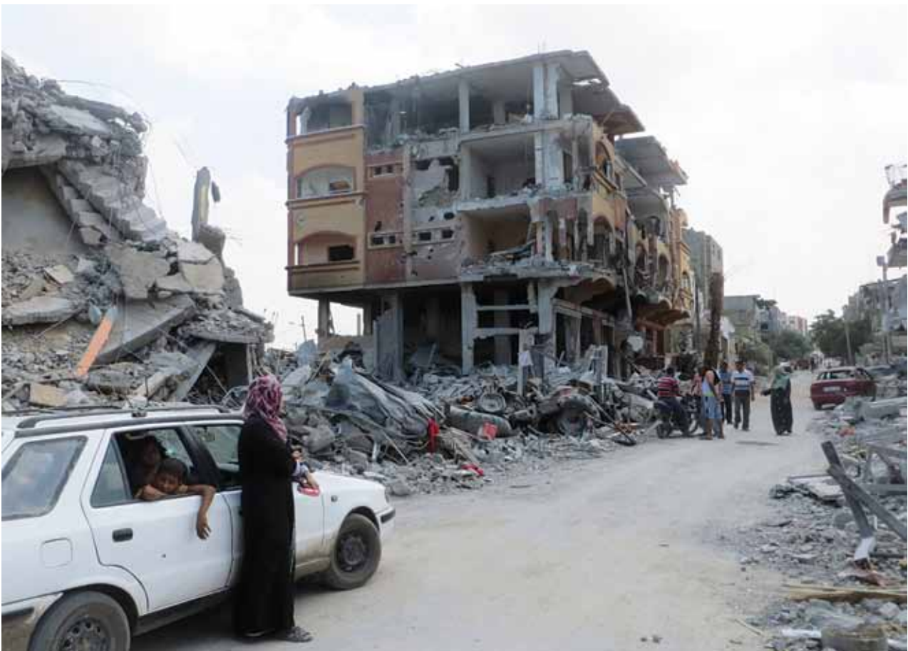
Damage to homes in Beit Hanoun.
