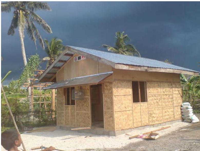
Working towards a total of 1,300, up to 1,019 houses have been built in Iloilo and Aklan, using techniques to enhance resistance to typhoons. Each completed house has an EcoSan latrine which provides options for market gardening and therefore, income generation. (Photo: International Federation of Red Cross and Red Crescent Societies)
