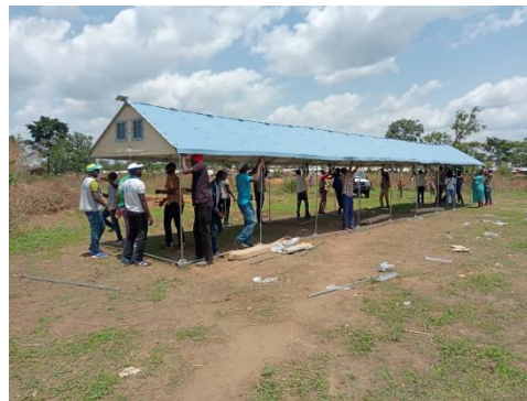
Pic 1 & 2 Setting up of the Refugee Housing Units, RHU, in Gado.
