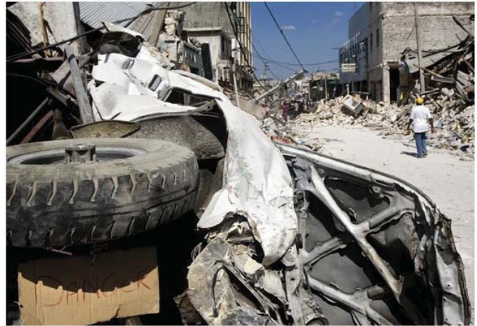
Haiti: Rubble of collapse buildings in downtown Port au Prince. Image: MINUSTAH- Marco Domino.©
