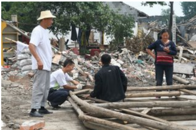
Villagers in Zundao township created temporary structures in anticipation that houses will not be reconstructed before winter. Photo: Francis Markus/International Federation
