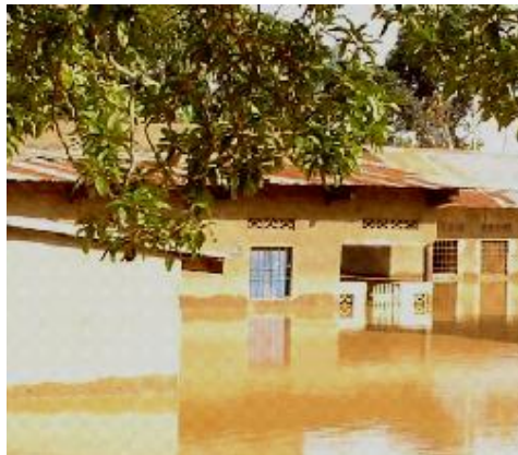
A view of a house that was flooded during the emergency phase.
