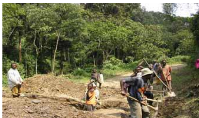
FAO road rehabilitation project in the North Kivu
