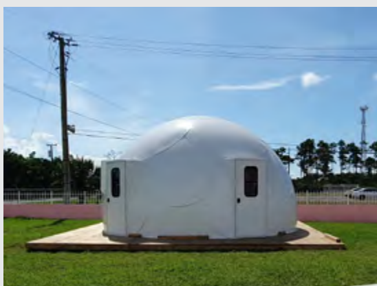
Sample Dome: NEMA Headquarters. Photo: John Marazita, October 2019.
