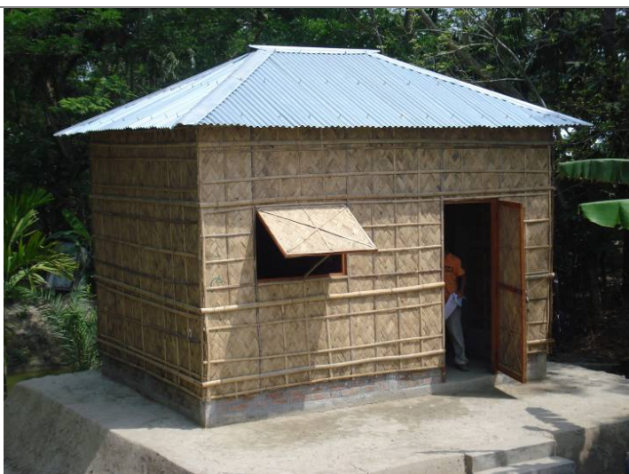
A residential core shelter built by the Cyclone Sidr operation in Bangladesh. 1,250 residential core shelters have been built by the Sidr operation.
