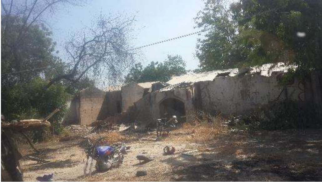
Destroyed buildings in “Doron Baga”
