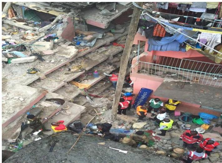
**Figure 1: 'Pancake collapsed building'. Photo. KRCS**
