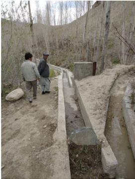
With support from USAID/OFDA, a Badakhshan village built this channel to direct floods away from homes and into irrigation canals (Courtesy of FOCUS).
